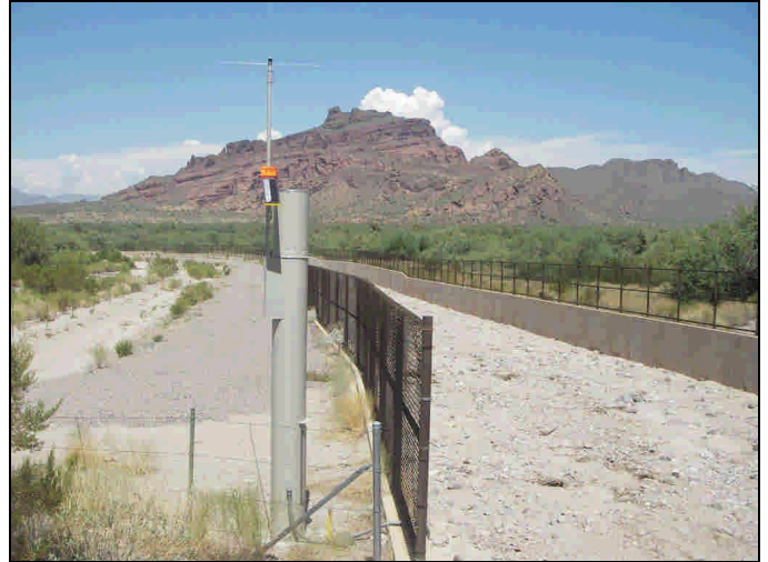
Water Level Station, Maricopa County
