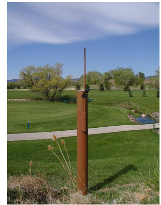
Packaged Pressure Transducer Station, City of Loveland, CO
